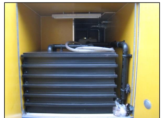
Aboveground Container-Housed Filter with Fresh Peat
